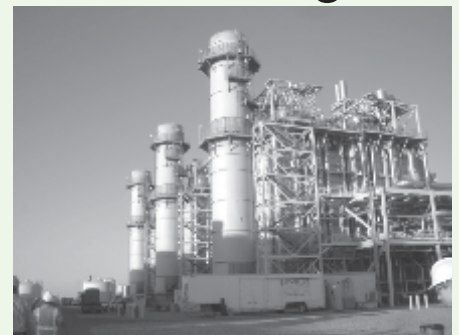
Above: HDPP's natural gas combustion turbine generator. This 3 Oxidation catalyst and duct burner helps reduce the facility's air emissions.
